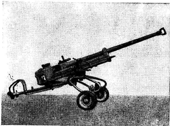
Figure 45.—Airborne version of 2.8 cm s. Pz. B. 41 (28/20-mm tapered-bore antitank gun).
