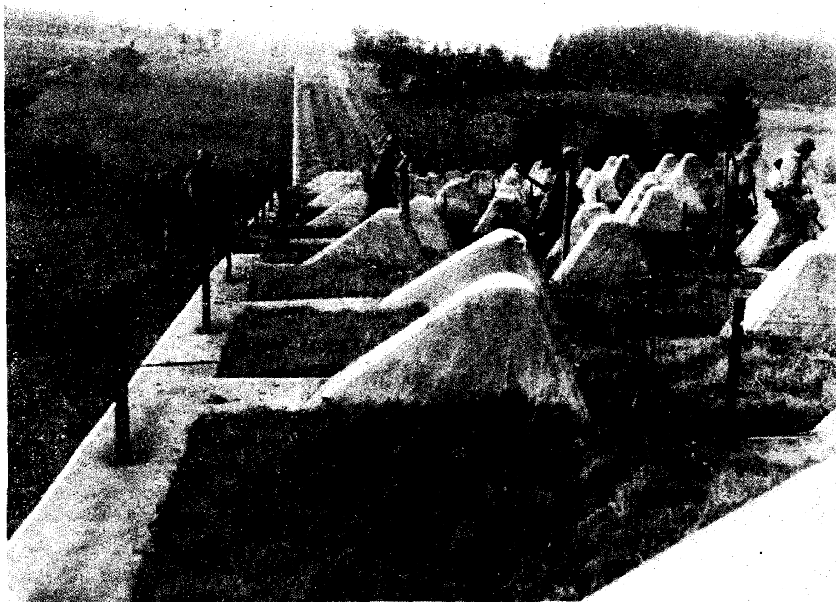
Figure 16.--Dragon's teeth showing concrete foundations.
