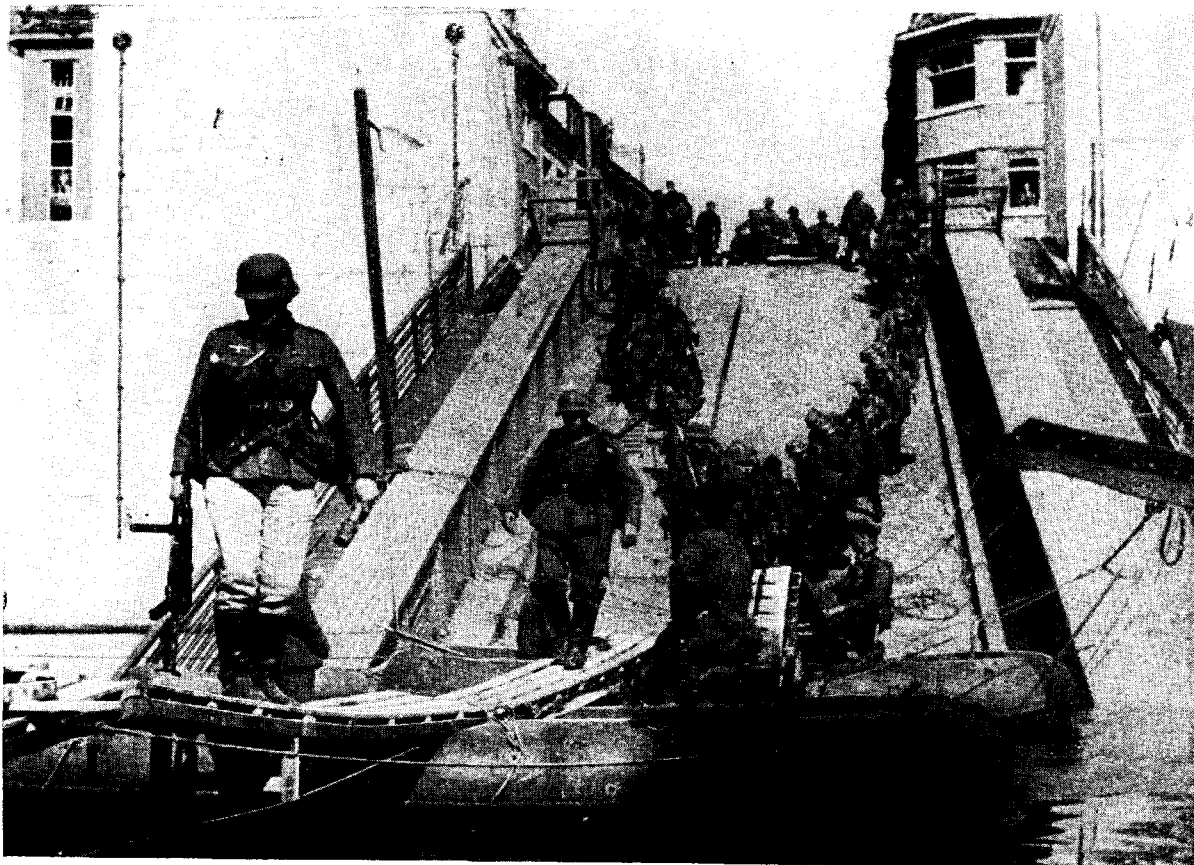
Figure 96.—Track bridge and medium pneumatic boat.
