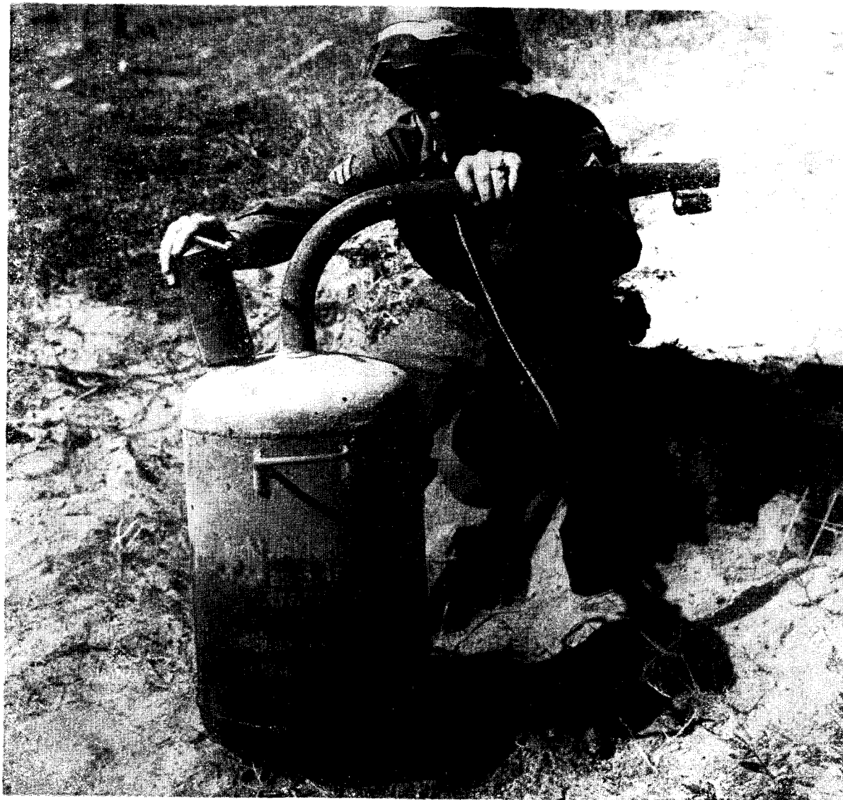
Figure 136.—German static flamethrower.
